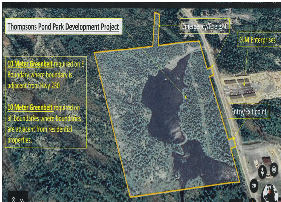
Figure 1. Thompson Pond RV Park Development Site
