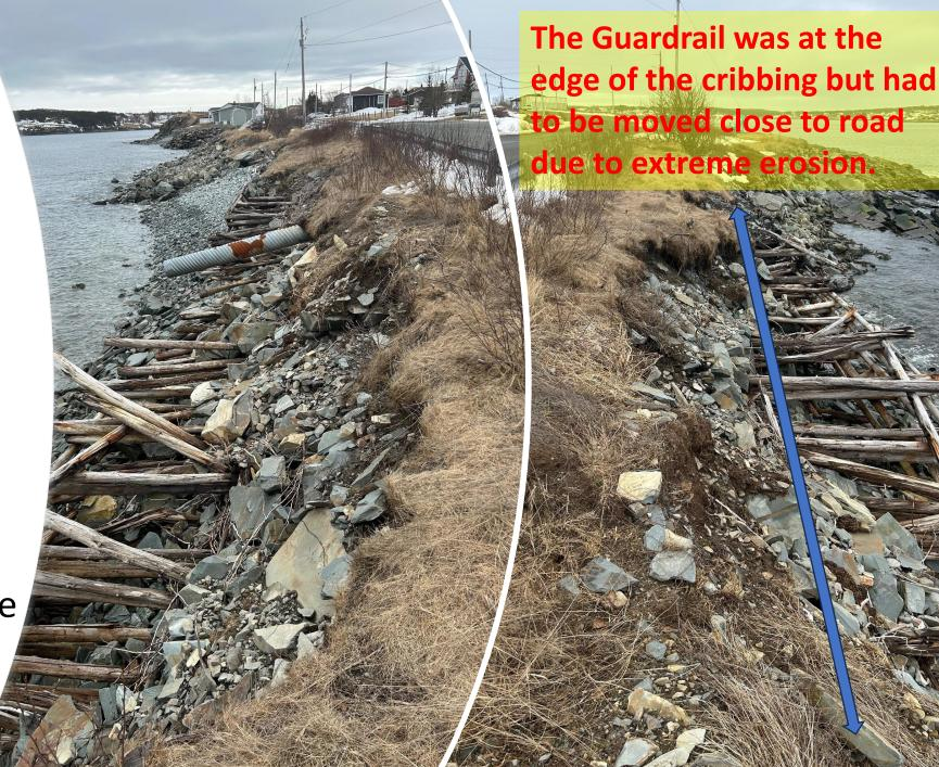
Shoreline severely eroded: approx. 15 to 20 feet completely gone Only about 5 feet of shoreline left before the road is damaged
